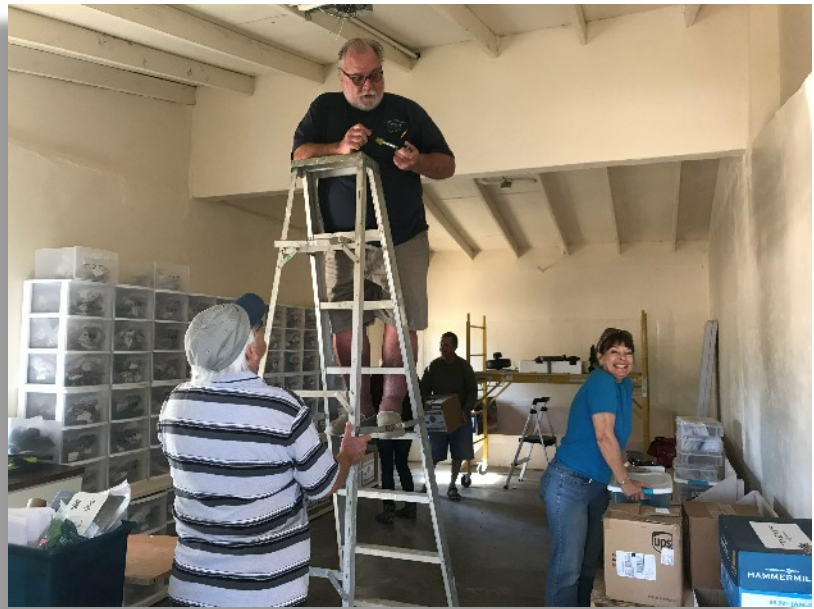
Richard Lenyk working on the electrical in the renovated optical clinic
